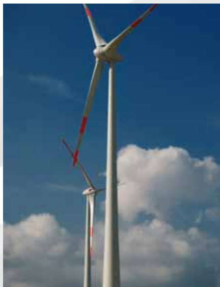
... Wind power units
