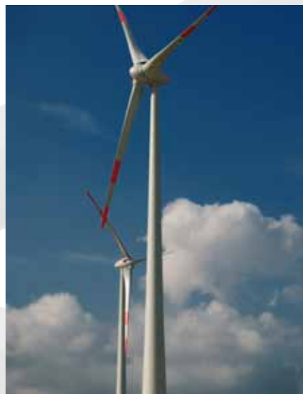
... Wind power units
